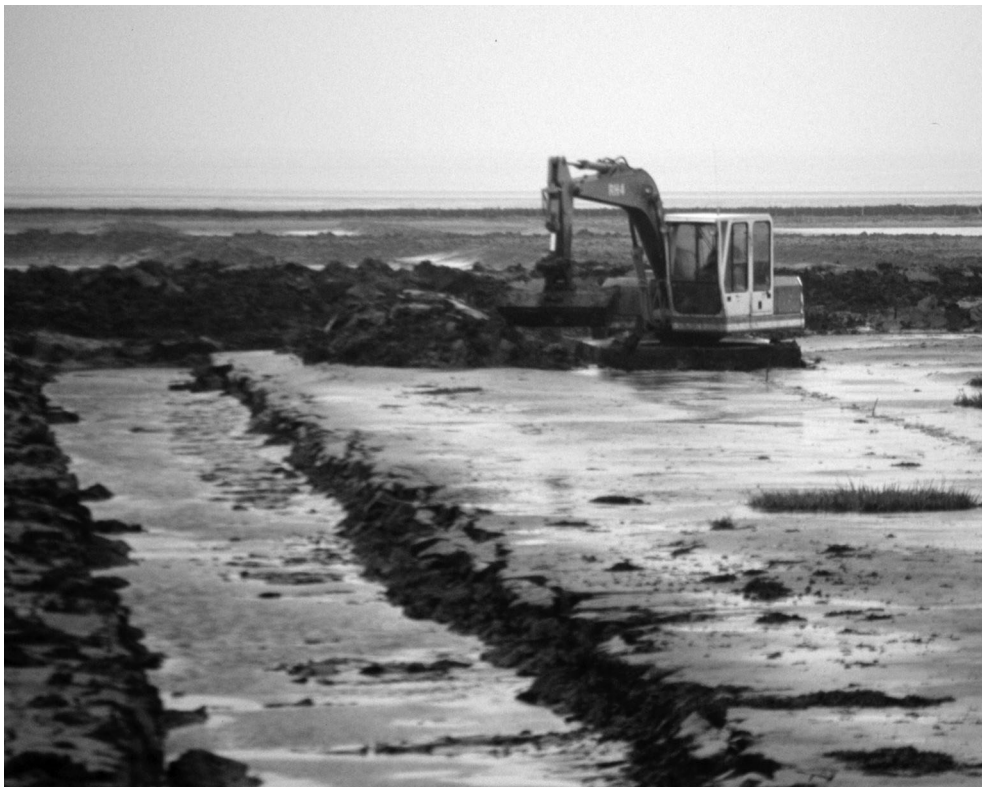
Figure 5. (a; top) Milling cutter in the Dutch sector of the Wadden Sea (note that the material from the ditch is evenly distributed on the flats). (b; bottom) Dredging machine in the Schleswig-Holstein sector of the Wadden Sea (note the huge piles of material left between the ditches).
