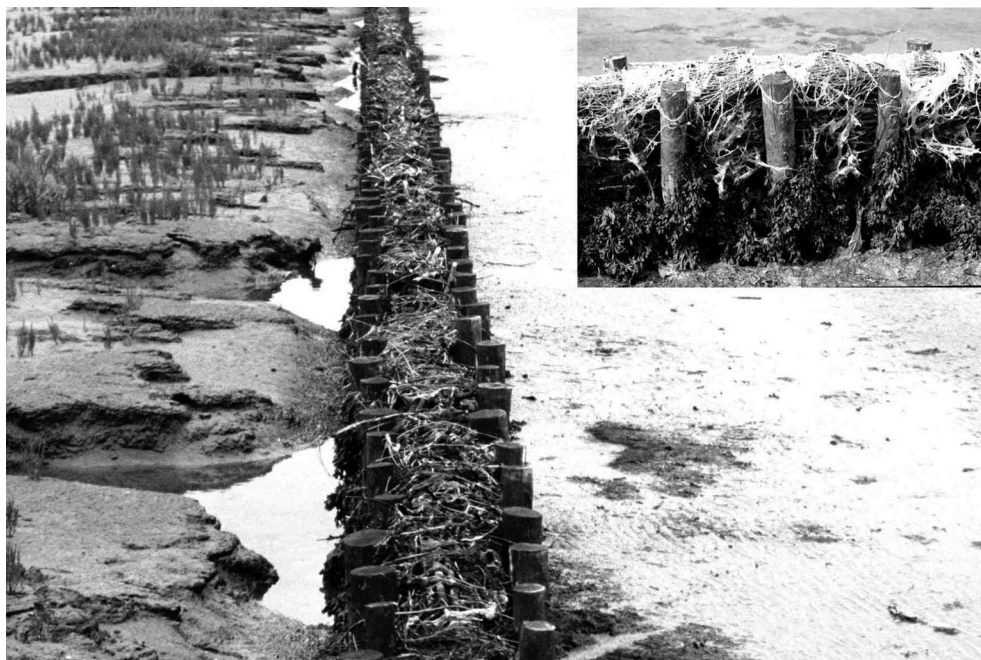
Figure 7. Brushwood groins in the Schleswig-Holstein sector of the Wadden Sea (the sea is to the right).
