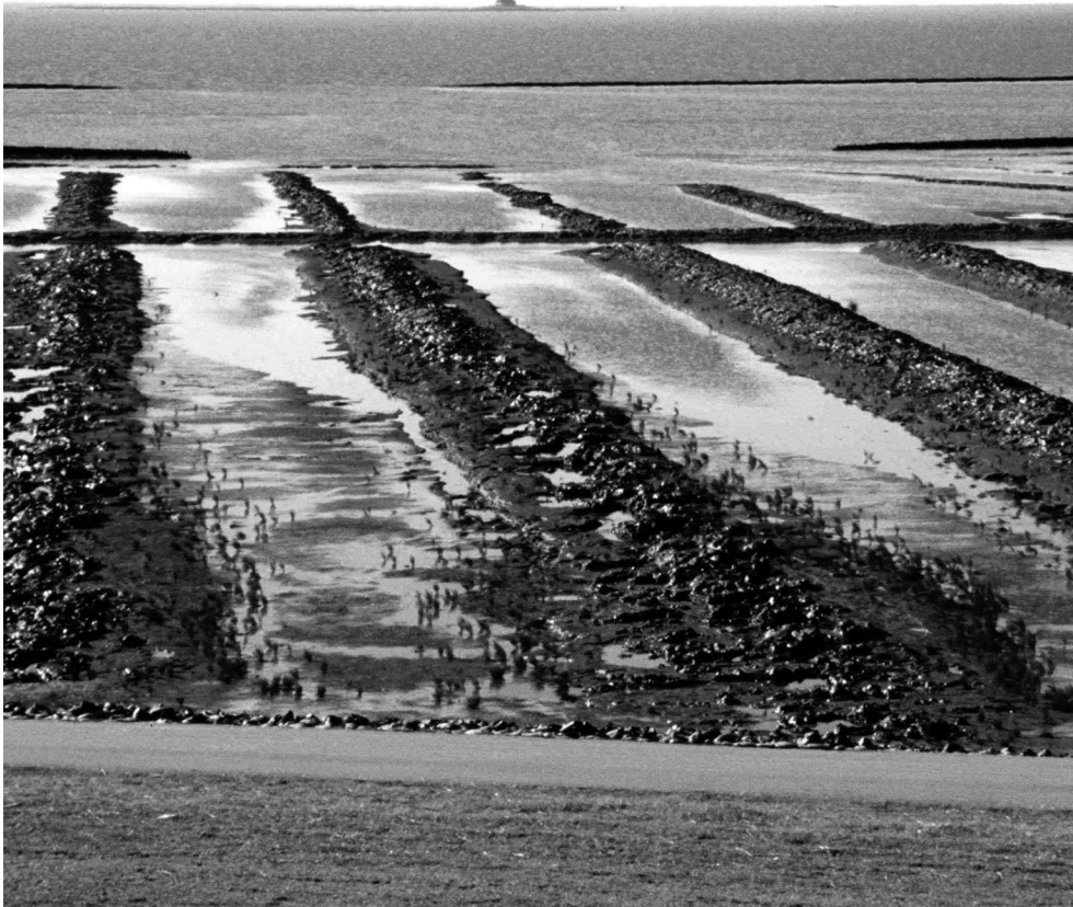
Figure 6. Drainage ditches in a groyn field in the Schleswig-Holstein sector of the Wadden Sea.
