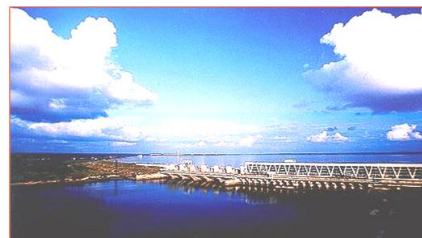
Fig. 9. Riga HPP Reservoir
