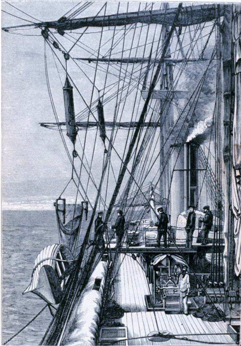
FIG. 17.—The Dredging and Sounding Arrangements on board the 'Challenger.'
